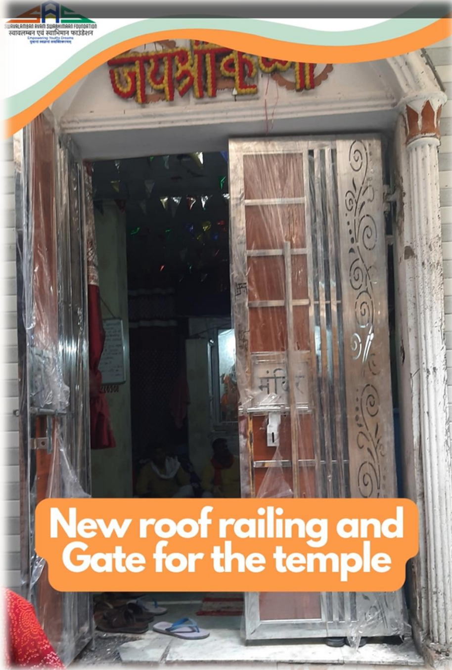
Figure 36 Temple Renovation @ Shiv Mandir Palam (Jul '25)
